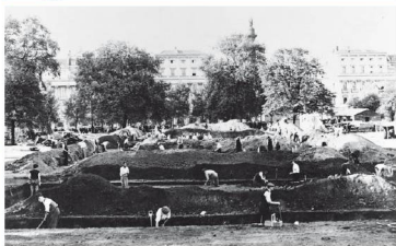
Digging air raid defences in London, September 1938.
